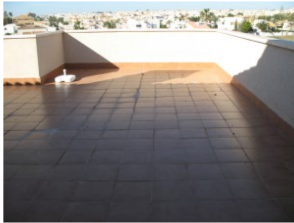
Roof Top Solarium
